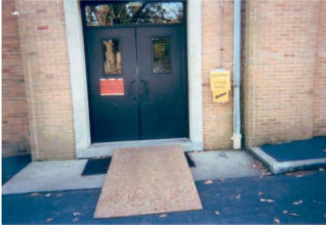
2. The main entrance does not allow the necessary 5 feet of level area on the outside of the doorway.
