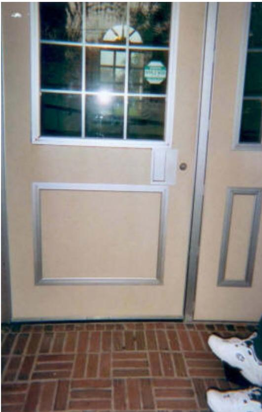
2. Door handles at main entrance not in compliance. Door handles should be easy to use without requiring tight grasping or twisting of wrists to open.
